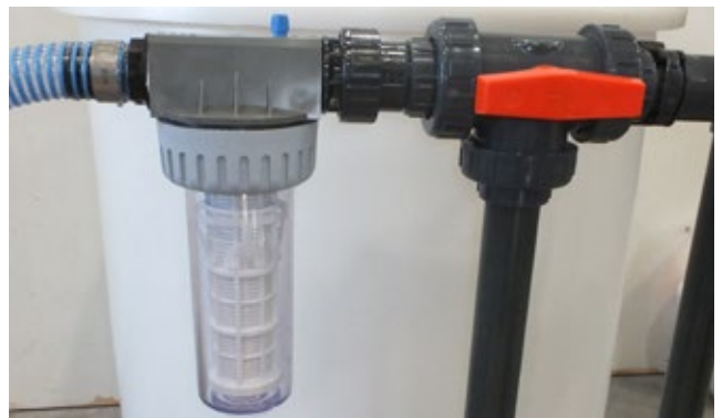
Heavy duty filter and 3-way valve
